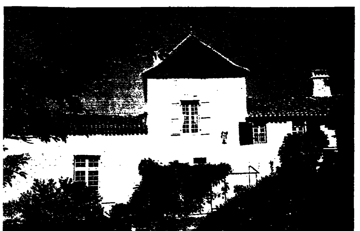
Restored: in Lot-et-Garonne is Gervésie, an old farmhouse/chateau with a tower block and large yard containing a 17th century dovecote
